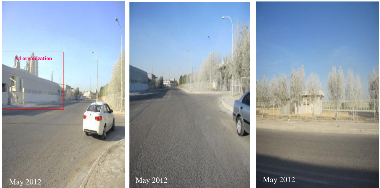
Figure 4.1: Environmental pollution continues one year after fines were imposed (photos: May 2012) a) the factory on white dust deposits in the immediate vicinity; b) trees further down the road are unaffected; c) the environment opposite the factory is covered in a layer of white dust.
