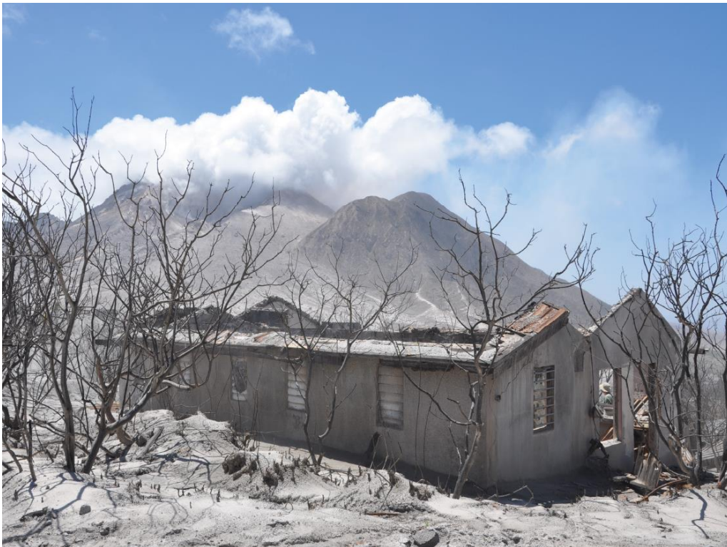
Figure 1.10: Example of one of the many badly damaged buildings in the exclusion area. Image taken in Streatham after 11 February 2010 dome collapse.
