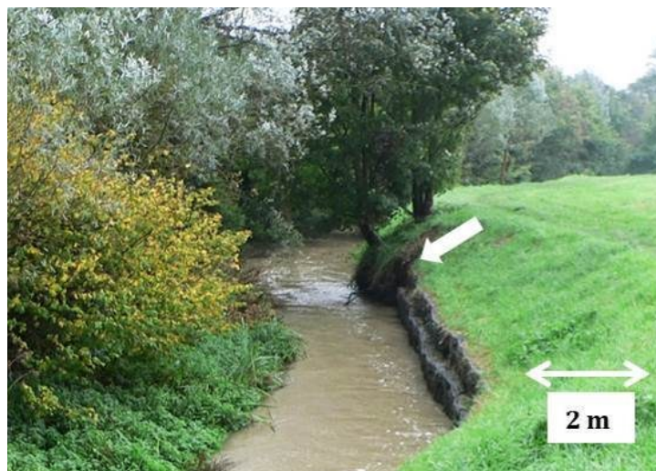
Fig. 2.5.3 Gabion revetment on the River Stour (Chapter 1, Fig 1.1.1). The arrow points to the location of a large scour at the end of the revetment. Note also the sliding tree that is falling into the channel.
