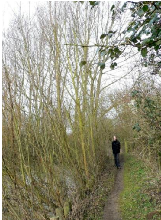
Fig. 4.1.6 Successful willow spiling approximately 15 years old on the River Ives in Bedfordshire.
