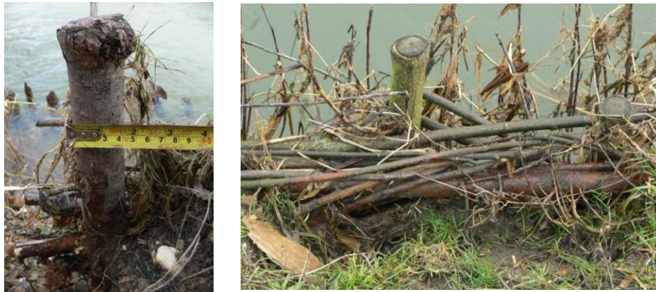
Fig. 5.4.15 Eroded backfill on the lower tier at the non-cohesive site in March 2010 with visible roots and woven part of spiling that was originally under the backfill.
