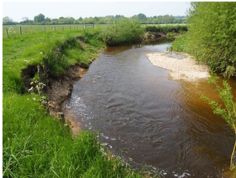
Fig. 7.2 Willow spiling at N1 site in Nayland on the River Stour in June 2012, looking upstream. Some dead stakes and scouring are visible on the left (right bank) and there is no growth from the revetment in the upper tier. On the other hand, a vigorous growth is seen from the shorter lower tier, in the top middle of the picture.
