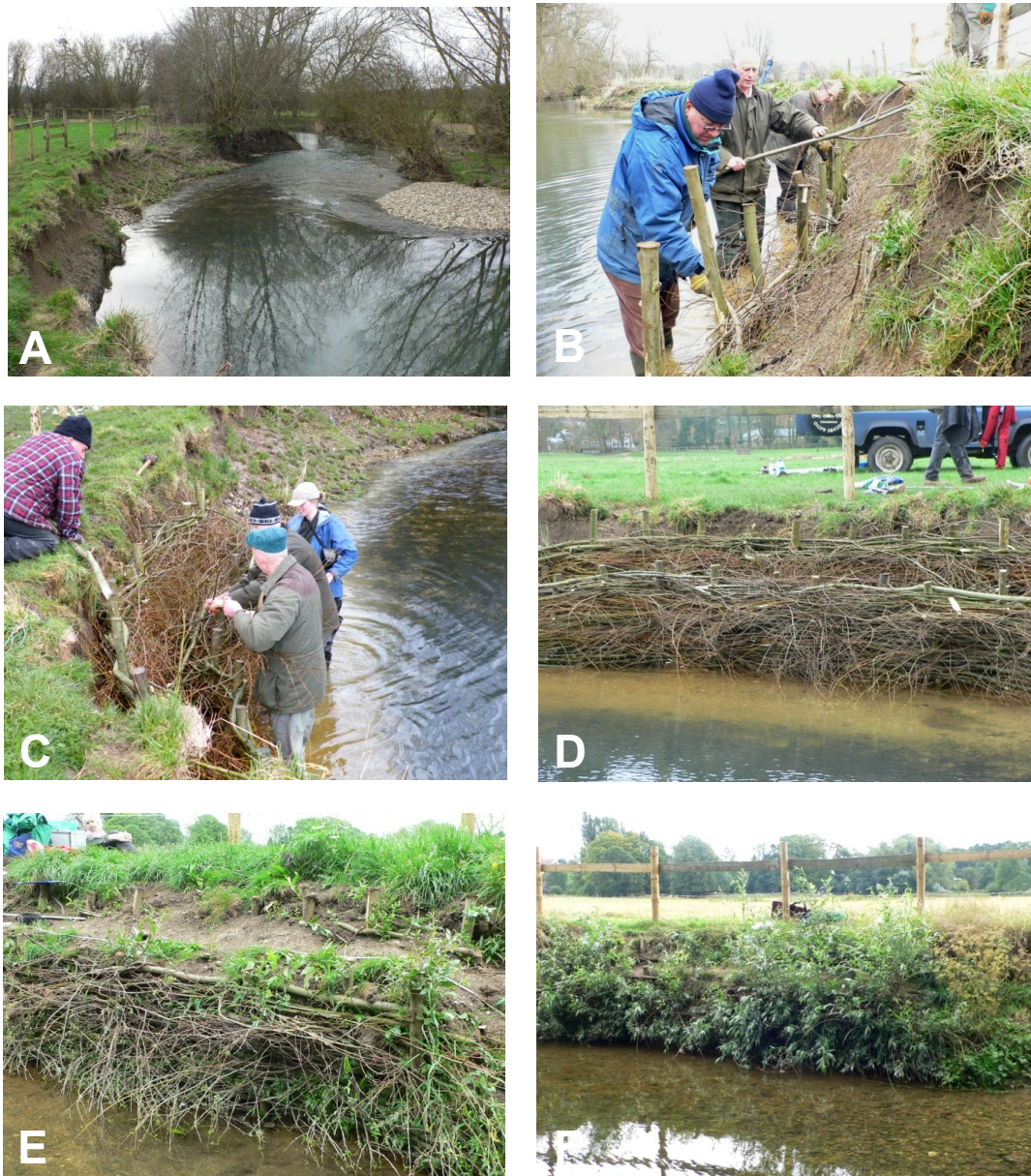
Fig. 5.2.1 Photographs from the project diary at the cohesive site in Sudbury S1: (A) site before stabilisation works, looking downstream; (B) Sudbury Common Lands volunteers weaving the lower tier; (C) finishing the weaving on both tiers; (D) completed spiling before backfill – all March 2009; (E) finished backfilled spiling with first shoots appearing - May 2009; (F) summer growth on the spiling, viewed from the right bank - August 2009.
