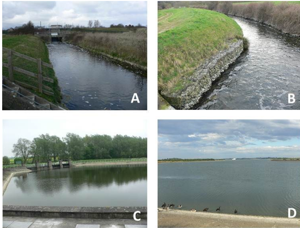
Fig. 3.1.7 The Stour part of the Ely Ouse to Essex Water Transfer Scheme (EOETS): (A) Outfall from the Kirtling pumping station, looking upstream; (B) Kirtling channel with weirs taking the water down to the River Stour, looking downstream, (C) Wixoe pumping station hexagonal reservoir and (D) The Abberton reservoir.
