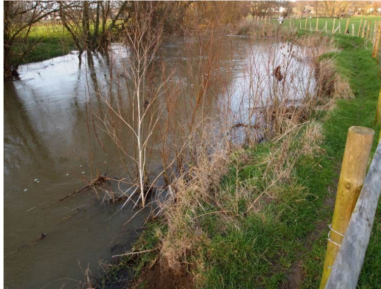
Fig. 7.1 Willow spiling in Sudbury at the S1 site on the River Stour, during a high flow event, looking upstream in March 2012. The spiling acts as a flow deflector and a trap for small floating debris and sediment.
