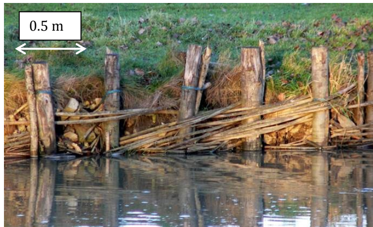
Fig. 4.1.5 Disintegrating spiling structure two years after installation on the River Great Ouse, Bedford, East Anglia.
