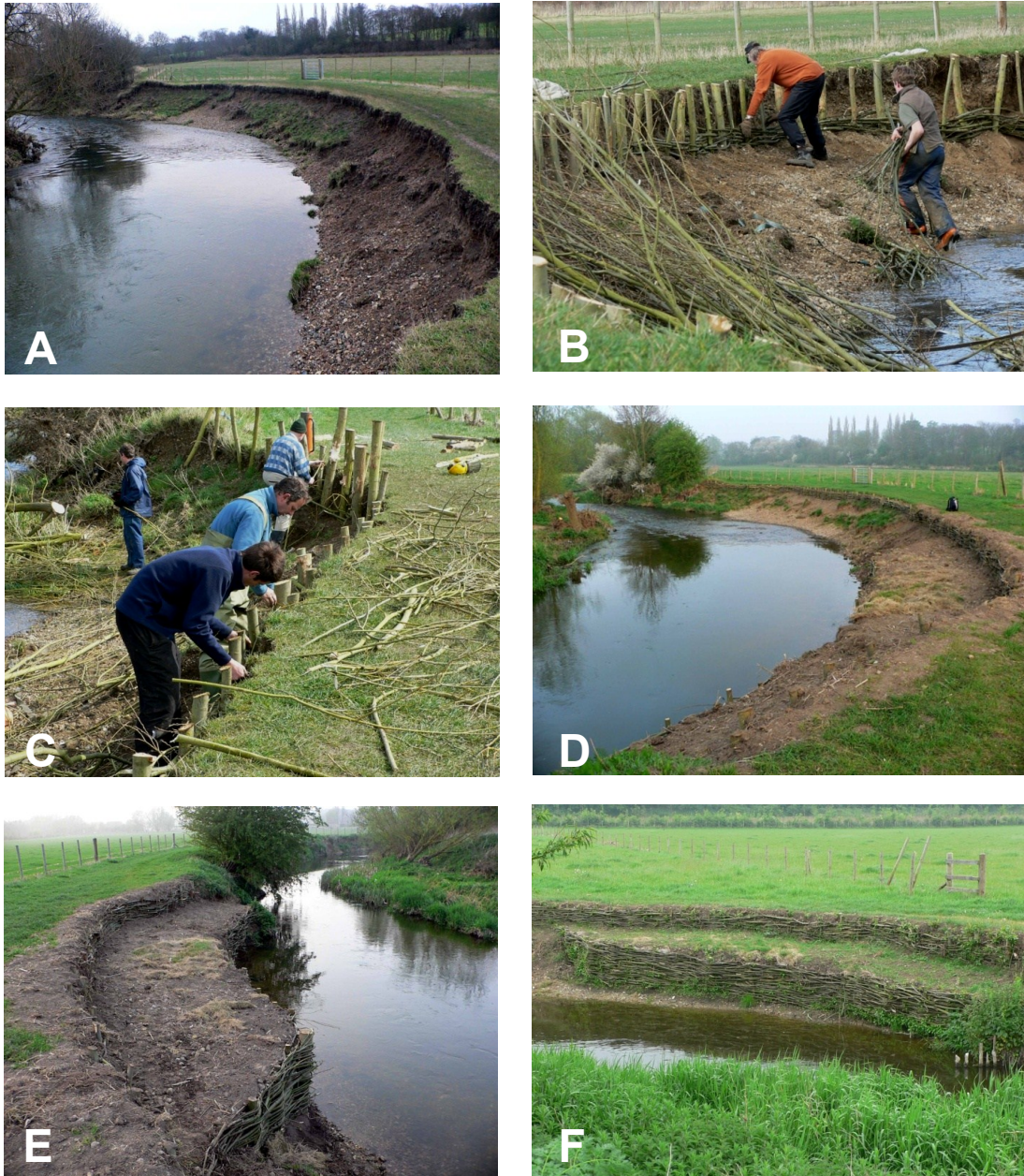
Fig. 5.2.2 Photographs from the project diary at the non-cohesive site N1 at Nayland: (A) project site before the works, downstream view - December 2008; (B) and (C) volunteers and landowner's staff weaving in the eroding gravel bank - March 2009; completed works: (D) view downstream and (E) upstream - April 2009; (F) spiling with first growth - May 2009.
