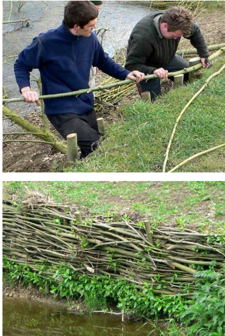
Fig. 4.1.1 Installation of willow spiling at N1 site in Nayland, March 2009 and the completed willow spiling wall with the initial growth, May 2000 (see location map on Fig. 3.1.1).
