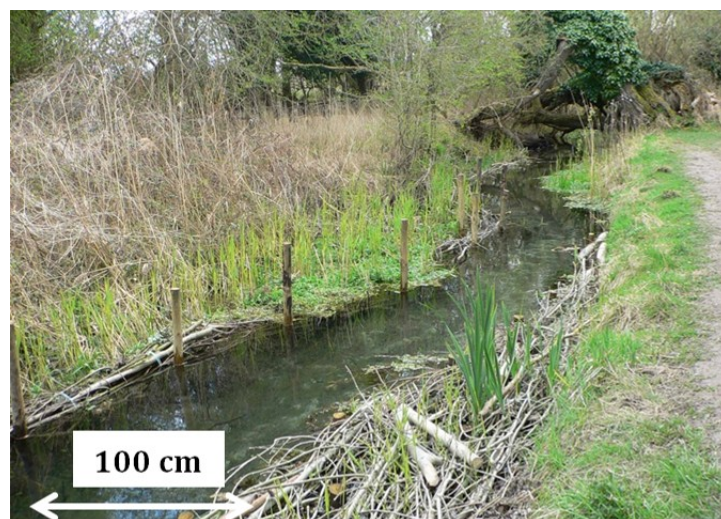
Fig. 2.5.1 Revetment using willow stakes, hazel faggots and reeds for river narrowing and habitat improvement, the River Shep, Cambridgeshire (TL384473), April 2008.
