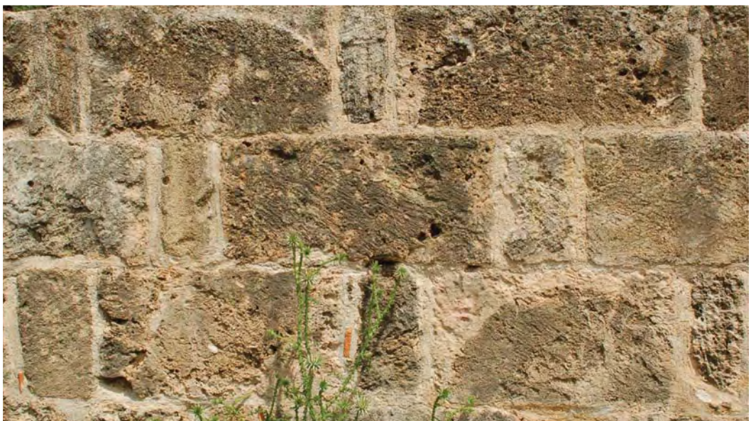
12.4 Wallwork. South outer wall. Detail
