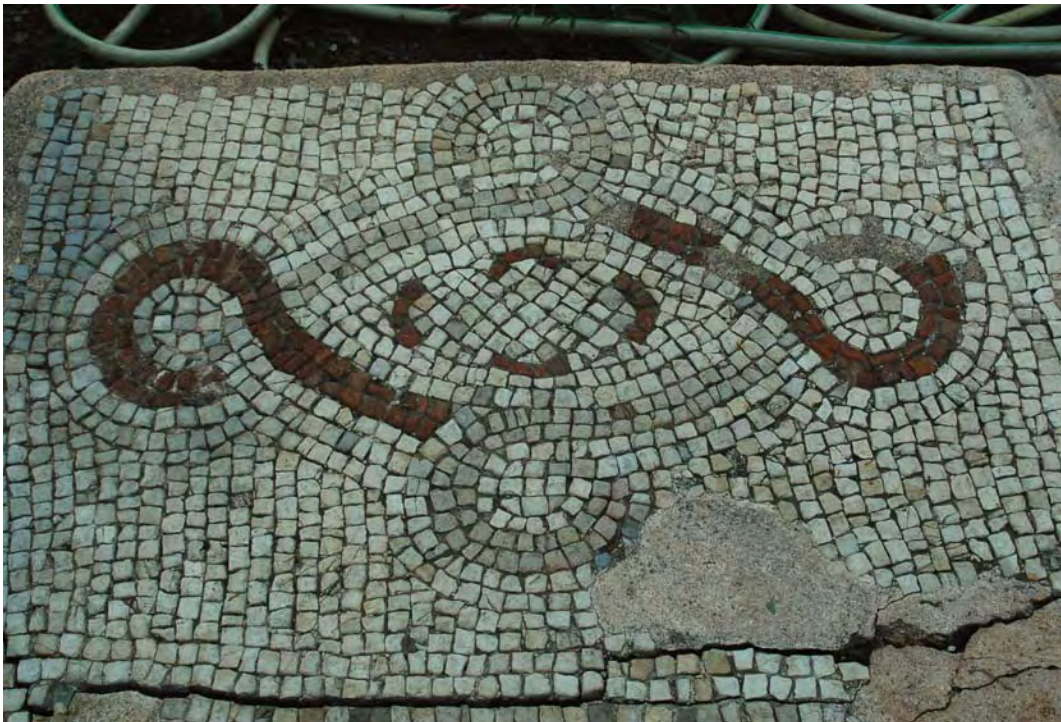
5.6 Threshold at north end of narthex looking south
