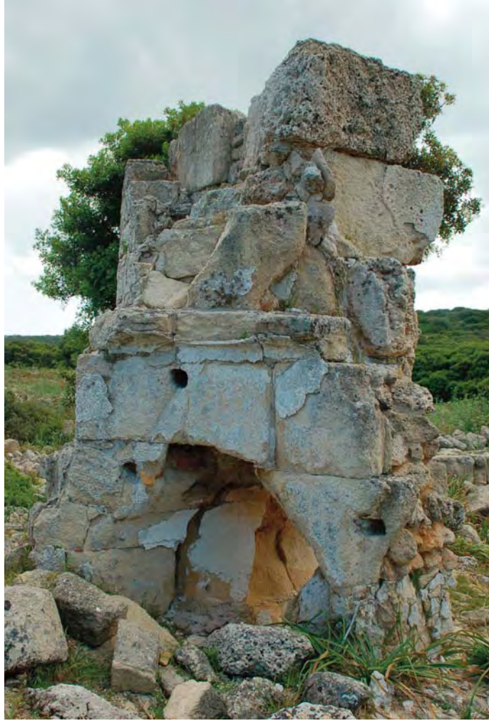
12.8 Southeast quadrant of north apsidiole with intersidal passage, looking southeast
