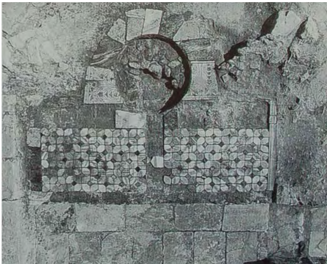
6.12 Paving of apse of north annex
