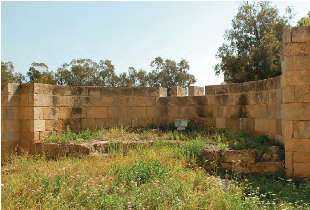
60.4 Central apse looking east
