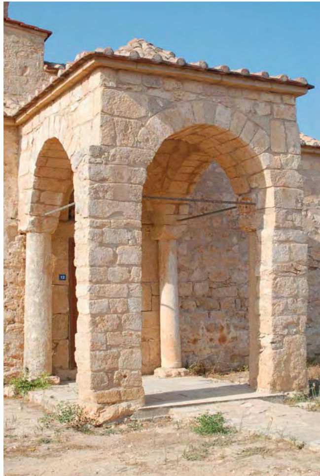
40.3 Porch looking northeast
