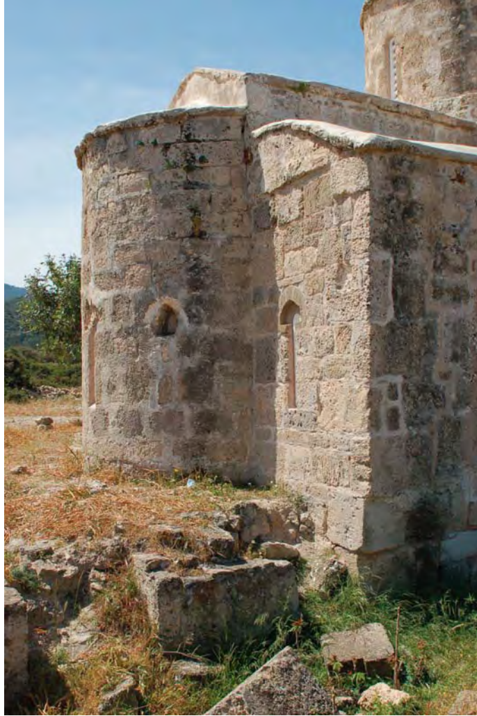
2.1 East end of Middle Byzantine church looking southwest
