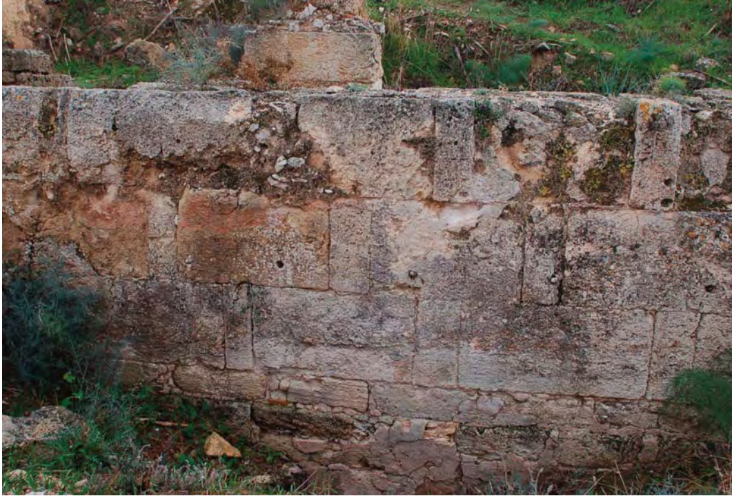
59.3 Header and stretcher wallwork. Inner wall of south aisle
