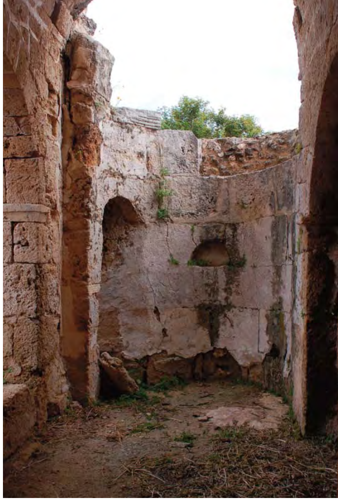
11.11 South aisle looking east
