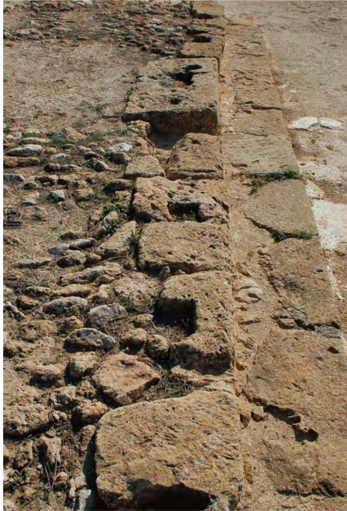
51.8 Sockets for chancel screen posts. Bema, western edge, looking south
