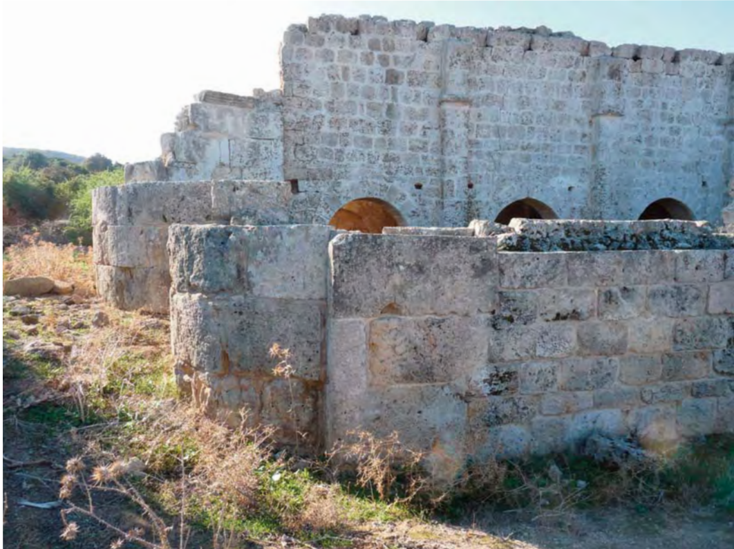
11.3 East end looking south
