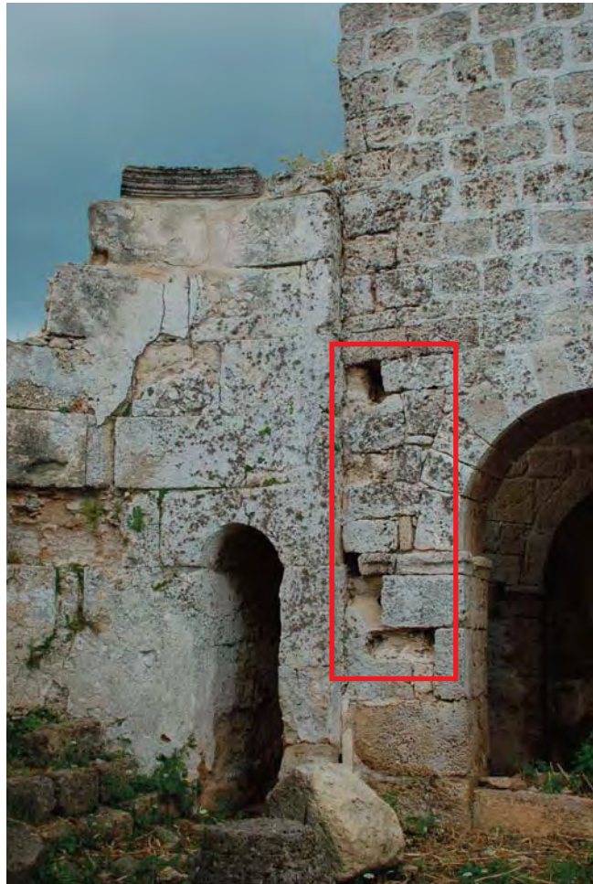
11.6 Junction of south wall of nave and apse. Embedded demi-shaft
