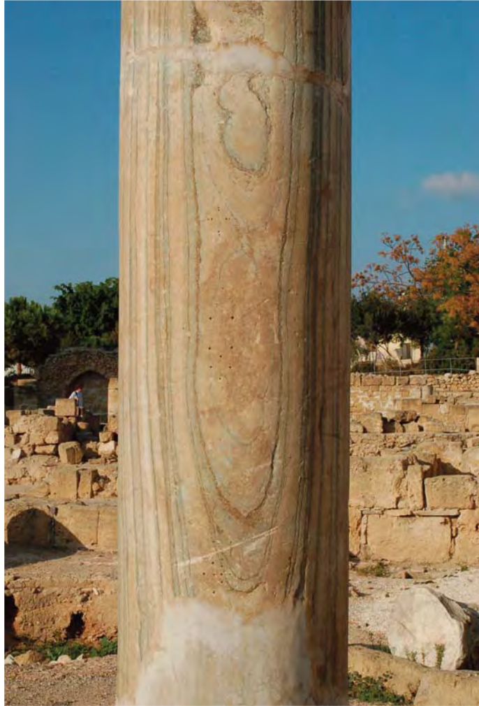
47.5 Cipollino column from south colonnade. Drill holes probably marking the position of crosses
