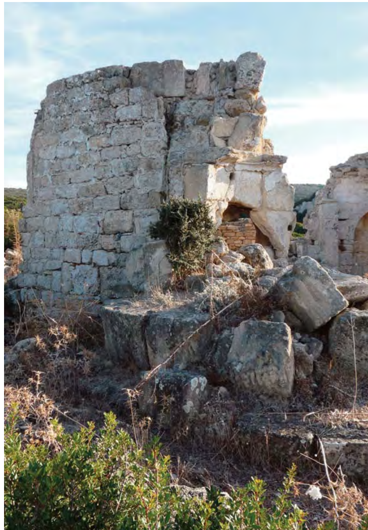
12.7 North and central apses looking south
