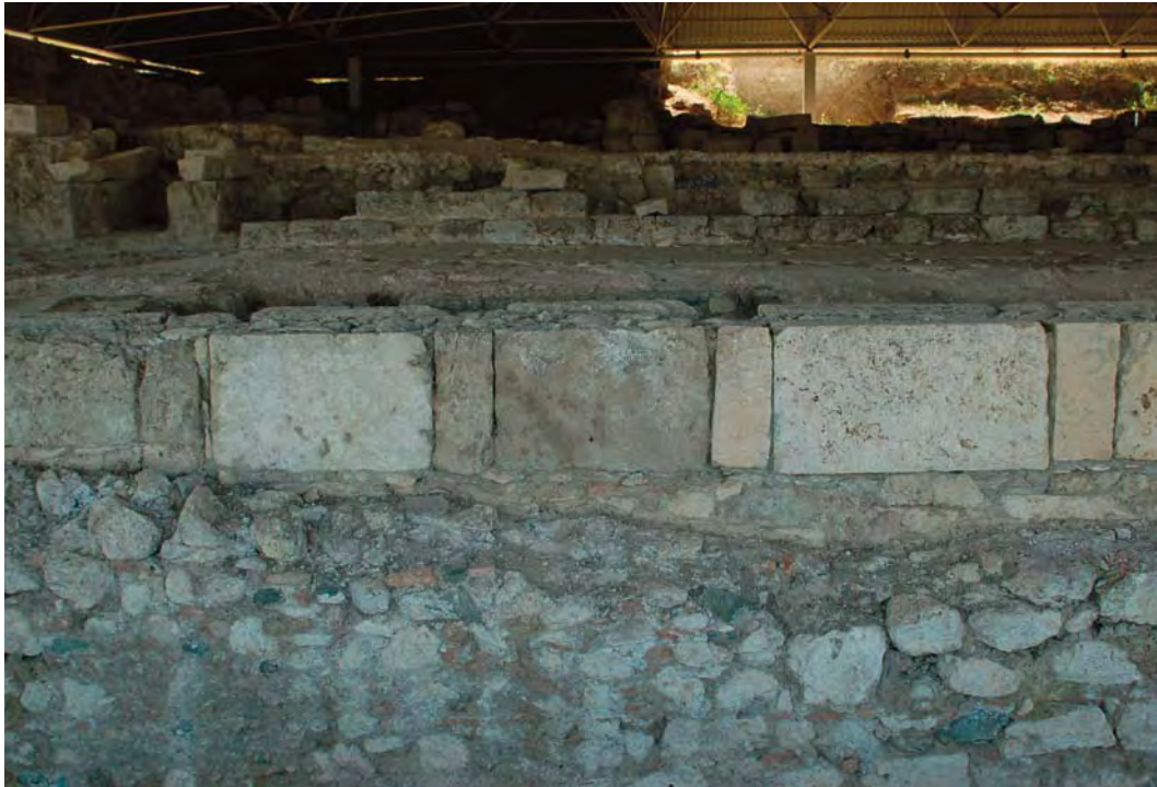
64.21 Basilica B. Header and stretcher wallwork on the north side looking south
