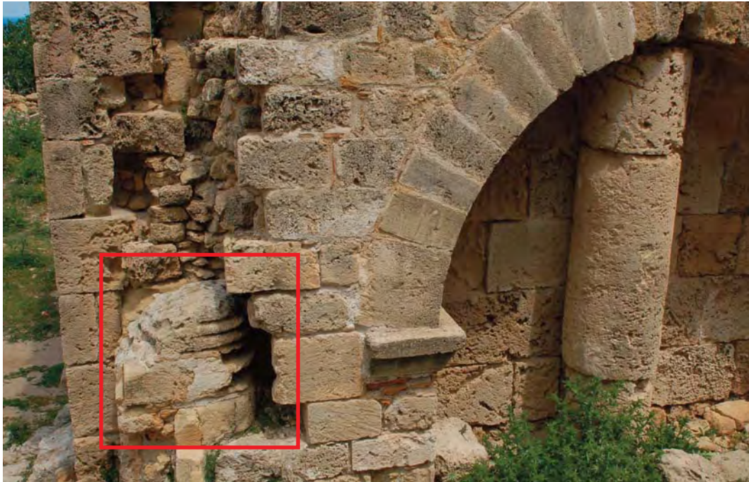
12.3 Embedded demi-column. East end of south colonnade, looking northeast
