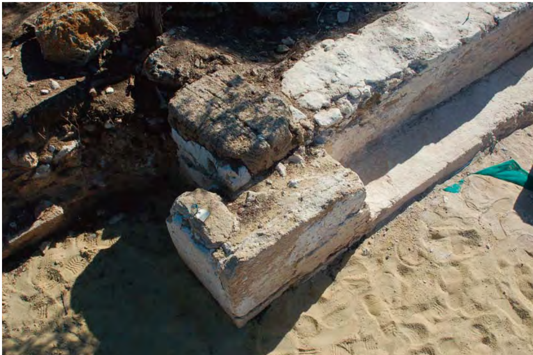
3.9 Clasping buttress. Junction of south aisle and south transept arm, looking southeast
