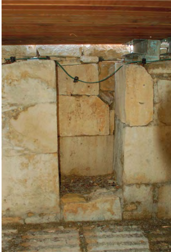
7.3 Rectangular niche in west wall of corridor
