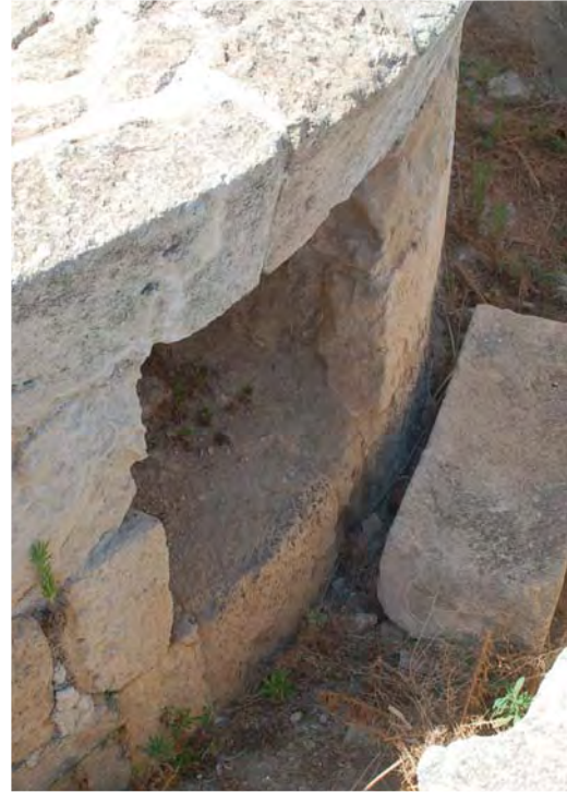
61.13 Axial recess in kyklion looking north
