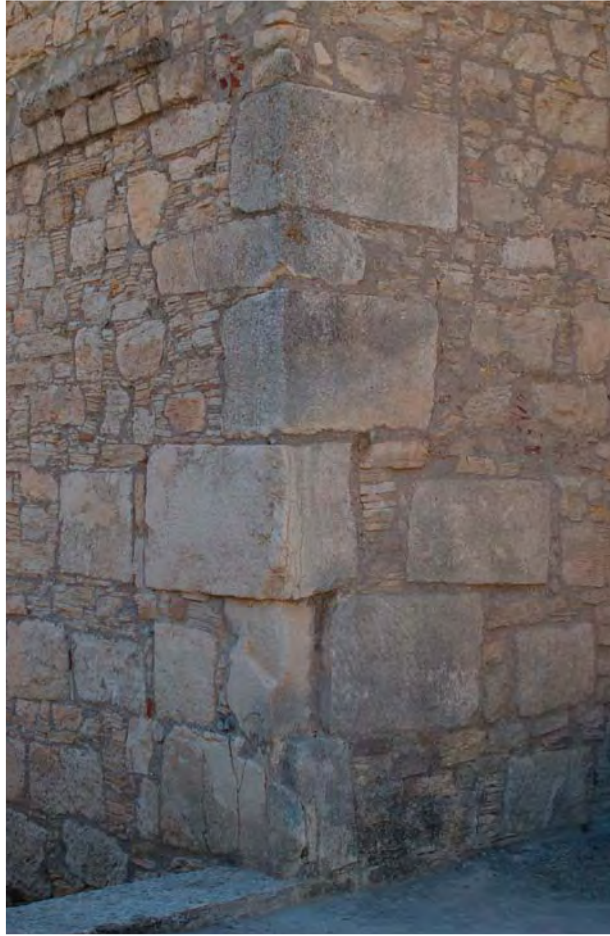
13.1 North east corner of later basilica
