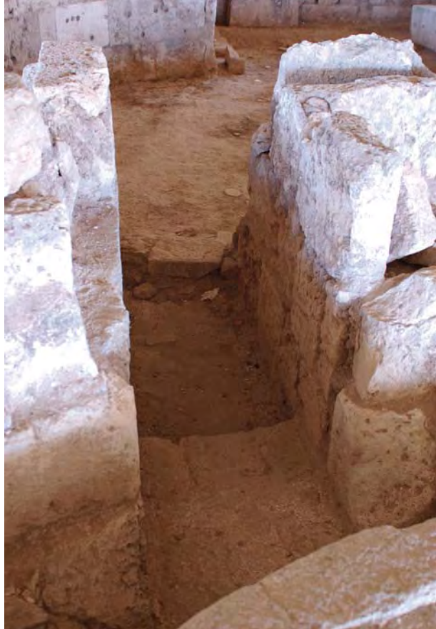
64.17 Basilica B. Passage between the central apse and the south apsidole looking south
