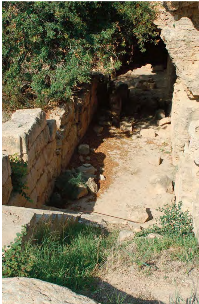
50.4 Subterranean passage at the eastern limit of site looking north
