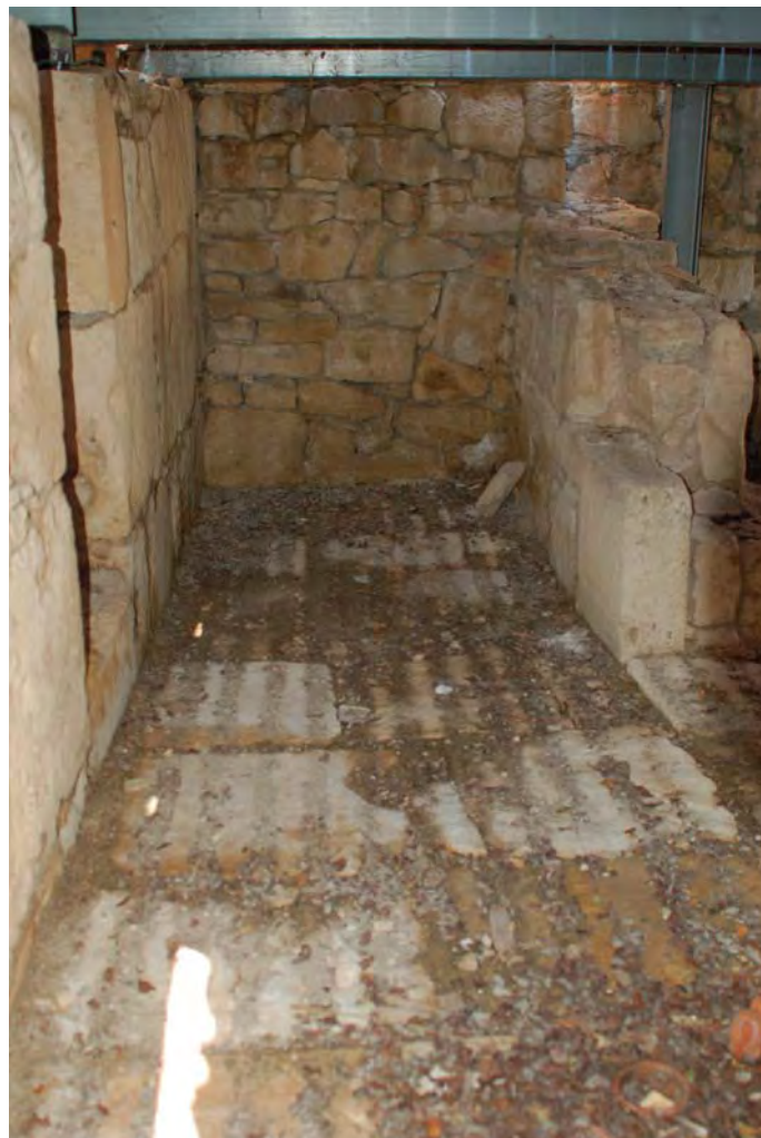
7.2 Corridor looking north
