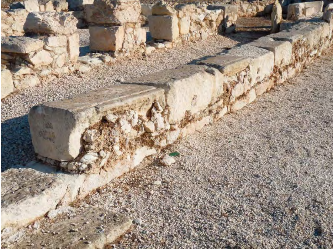
33.3 Reused seating in the north wall looking northeast
