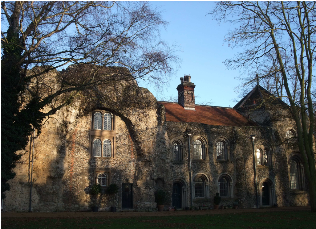
Fig. 61 The remains of the west front of the abbey church, Bury St Edmunds
