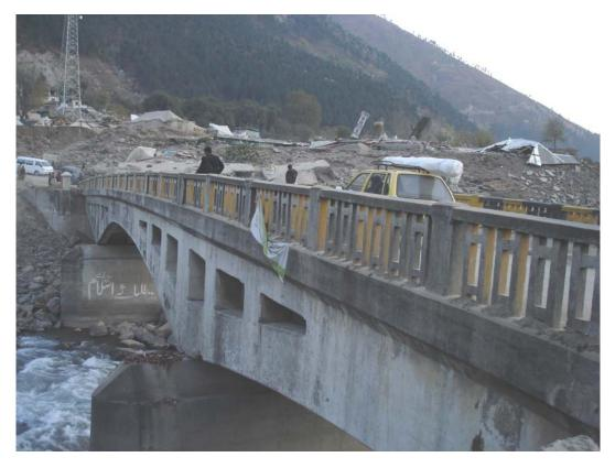
Figure 5.1: Laterally displaced RC deck of the vehicle bridge in Balakot
