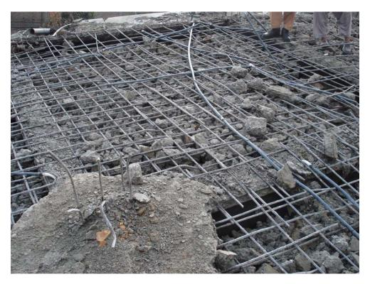
Figure 3.45: Reinforcement layout of a collapsed slab revealed after removing the concrete
