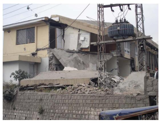
Figure 3.4: Damaged 2-storey concrete block masonry building in Muzaffarabad
