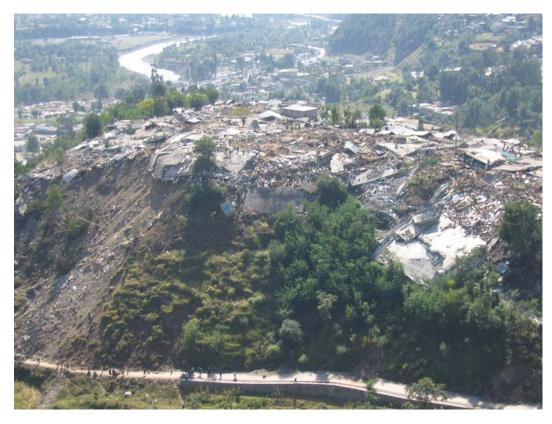
Figure 3.12: Collapsed and extensively damaged concrete block URM residential units in zone 1 overlooking Balakot city centre (photo by Kathrin Renner (Arup) and US Army)
