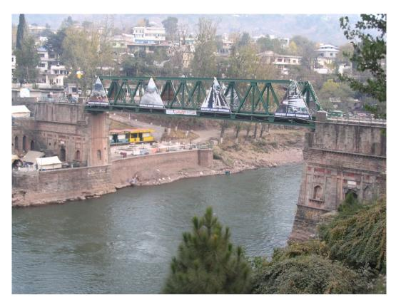
Figure 5.6: Undamaged pedestrian bridge across Jhelum River, Muzaffarabad. Bridge consists of steel truss single span simply supported on brick masonry gravity abutments
