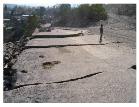
Figure 5.10: Ground cracks through a road in Muzaffarabad
