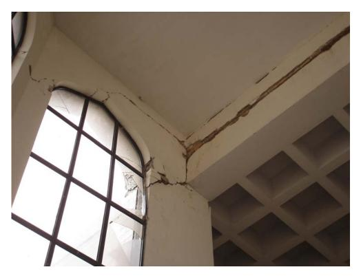
Figure 3.36: Shear cracks through the brick masonry column and roof beam connection at the Muzaffarabad Supreme Court building. Damaged glass due to shearing through the window
