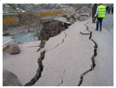
Figure 4.27: Retaining wall collapse leading to unstable pavement and road sections on a major route through Muzaffarabad
