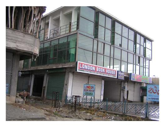
Figure 3.49: Permanent drift at ground floor due to soft-storey in RC frame and slab 3-storey commercial structure, Abbottabad. The ground floor drift prevented large deformation at upper floors, hence glass frontage was intact
