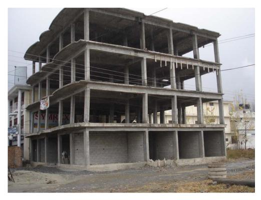
Figure 3.48: Permanent drift at the first floor of an RC frame and slab 4-storey commercial structure under construction, Abbottabad. Ground floor drift may have been prevented by the infill masonry walls
