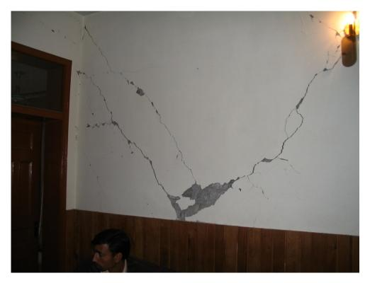
Figure 3.37: Diagonal shear cracks through the brick URM walls of the Muzaffarabad Tourist Information Office, moderate damage
