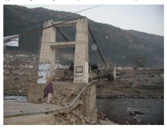
Figure 5.2: Pedestrian bridge with damaged approaches in Balakot
