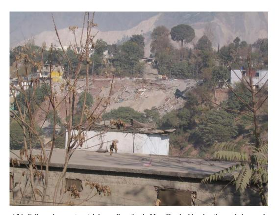
Figure 4.24: Collapsed concrete retaining wall section in Muzaffarabad leaving the road above vulnerable to further collapse
