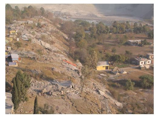
Figure 3.20: Collapsed stone and concrete block URM residential buildings on the hill and slight to moderately damaged residential buildings in the valley below. Collapse may be due to ridge effect or slope failure, Muzaffarabad
