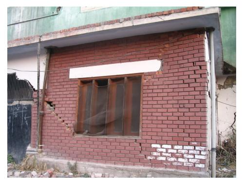
Figure 3.21: Diagonal shear cracks through window on a brick URM residential building, moderate damage, Muzaffarabad
