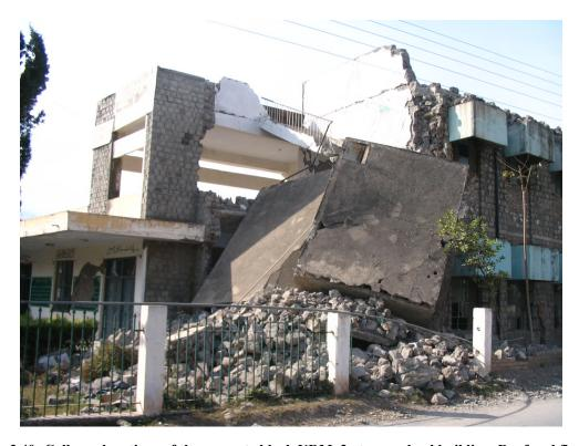
Figure 3.40: Collapsed sections of the concrete block URM, 2-storey school building. Roof and floor slab collapse due to failure of masonry bearing walls, Muzaffarabad
