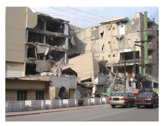
Figure 3.32: Collapsed section of Samgam Hotel, RC frame and slab construction, 5-storey. Collapse due to failure at beam/column connections, Muzaffarabad
