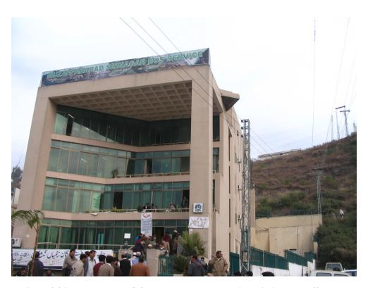
Figure 3.34: Undamaged RC frame and slab commercial building, Muzaffarabad
