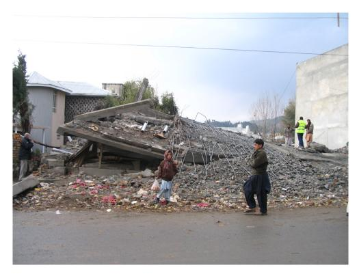
Figure 3.43: Collapsed RC 3-storey commercial and residential building. Collapse appears to be due to failure of beam/column connections, Abbottabad
