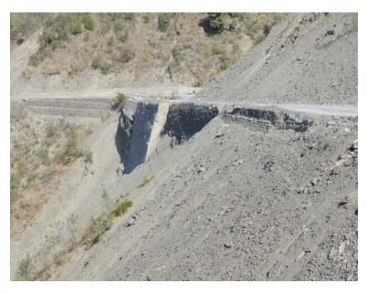
Figure 4.33: Road network and topography: reactivated landslide blocked this road for about 24 hours and has started to undercut the abutment. View from the same position as Figure 4.32
