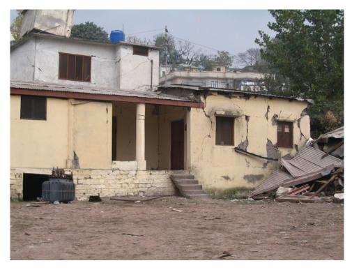
Figure 3.23: Shear cracks through the concrete block masonry wall of a residential building, moderate damage, Muzaffarbad
