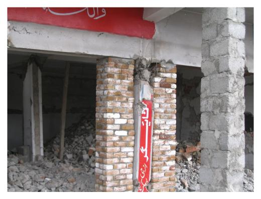
Figure 3.46: Extensively damaged 3-storey RC commercial building. Failed beam/column connections due to lack of shear or confinement reinforcement and inadequate layout, collapsed and cracked brick masonry infill walls inside the building, Abbottabad
