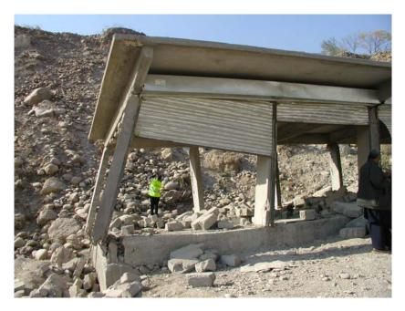
Figure 4.31: Rock falls and showers. Cobble and boulder material on slopes showered down on road transport during the earthquake. This site in Muzaffarabad City is above and behind the cracked road edge visible in Figure 4.5
