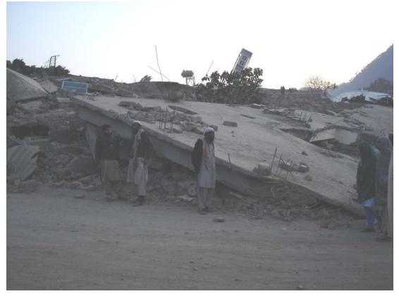
Figure 3.17: Collapsed single storey RC frame and slab commercial/retail building in Balakot city centre
