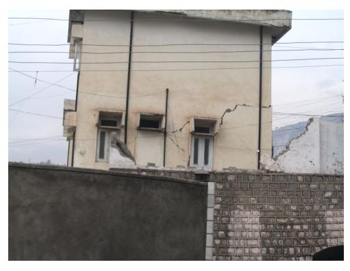
Figure 3.27: Diagonal shear cracks through concrete block wall of RC frame and slab commercial building with masonry infill walls, moderate damage, Muzaffarabad
