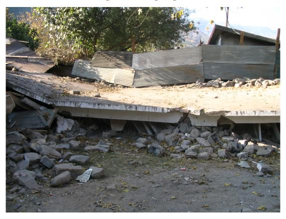
Figure 3.15: Collapsed concrete block URM residential building in Balakot
