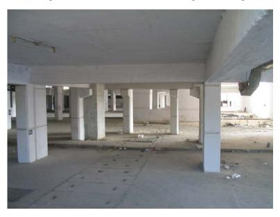
Figure 3.51: Soft-storey basement in a building adjacent to the collapsed building at Margalla Towers
