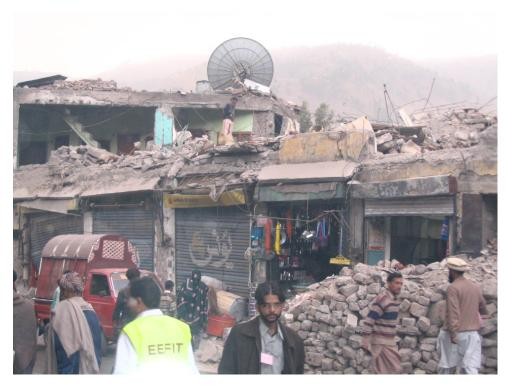
Figure 3.25: Collapsed roof of 2-storey RC frame and slab commercial buildings with concrete block masonry infill walls. Failure of beam/column connections at upper floor. Intact ground floor walls and first floor slab, Muzaffarabad
