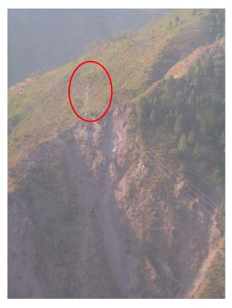
Figure 5.13: Potentially vulnerable transmission tower on the crest of a shallow depth landslide
