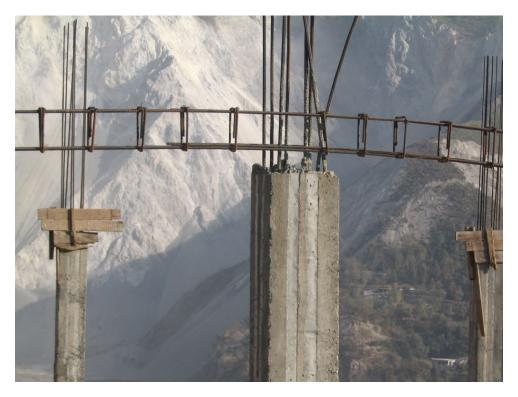
Figure 3.31: Incorrect splicing of reinforcing bar at beam/column connection of a moment frame under construction. Shear links configuration inadequate for seismic shear forces
