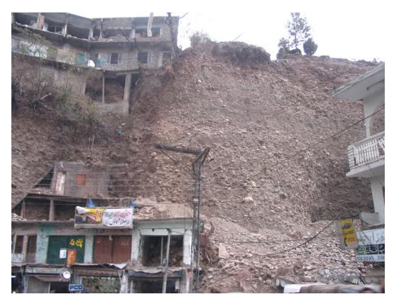
Figure 4.18: Slope failure burying and extensively damaging the commercial building below and destabilising the residential structure above, Muzaffarabad
