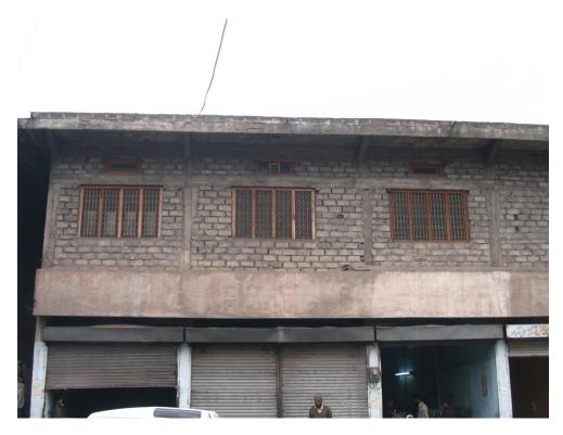
Figure 3.28: Undamaged RC frame and slab commercial building with concrete block masonry infill walls. RC lintel beam continuous over the structure perimeter, Muzaffarabad
