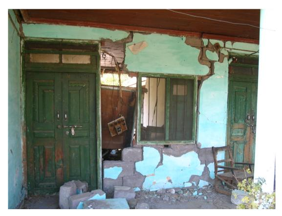
Figure 3.3: Damaged unreinforced concrete block masonry office building south of Balakot
