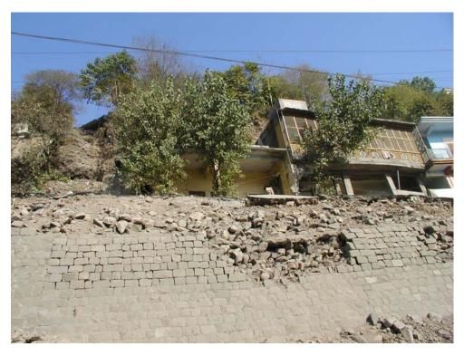
Figure 4.25: Stone block masonry retaining wall in Muzaffarabad: slippage and collapse of this wall undermined buildings
