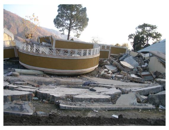
Figure 3.5: Collapsed unreinforced brick masonry house in Balakot
