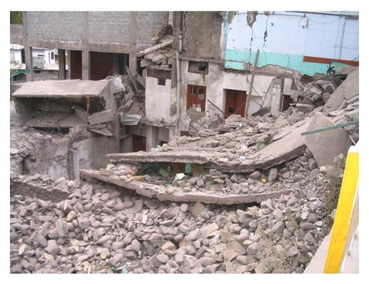
Figure 3.26: Collapsed 2-storey concrete block URM commercial building. Floor and roof collapse possibly due load bearing wall failure in shear and out-of-plane and high inertia loads from RC slabs, Muzaffarabad
