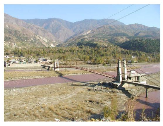
Figure 5.3: Undamaged pedestrian footbridge crossing Kunhar River on route to Balakot
