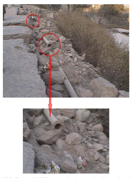
Figure 4.39: Smaller geotechnical failures: ruptured cast iron water pipe adjacent to the cracked and subsided road visible in the foreground of Figure 4.5
