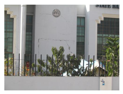
Figure 3.38: Shear cracks through the brick URM walls of the State Bank of Pakistan building, moderate damage
