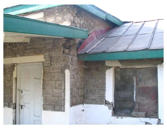
Figure 3.14: Cracks through stone and mortar in a stone URM building adjacent to the extensively damaged stone building in Figure 3.5
