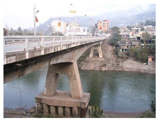
Figure 5.5: Undamaged vehicle bridge across Jhelum River in Muzaffarabad. RC bridge deck, multi-span with integral abutments supported on RC piles with steel casing
