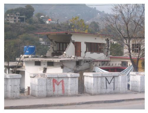
Figure 3.22: Partially collapsed upper floor walls of a 2-storey concrete block URM residential building with RC slab floors and roof. Shear and out-of-plane failure of concrete block bearing walls,
