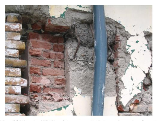
Figure 3.47: Example of failed beam/column connection due to poor shear and confinement reinforcement detailing
