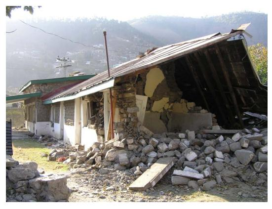
Figure 3.13: Extensively damaged stone URM building with metal roof in Balakot, used by the local audit officer
