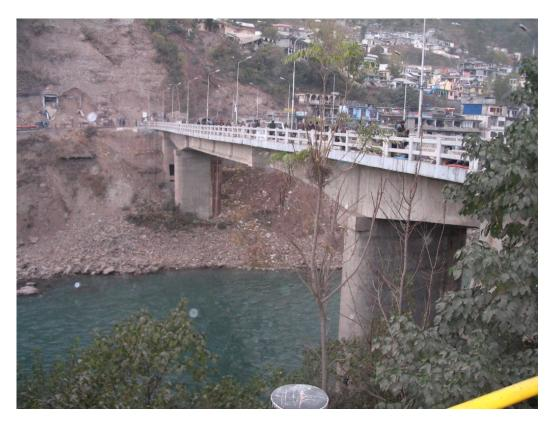
Figure 5.7: Undamaged vehicle bridge across Nelum River, Muzaffarabad. RC spans simply supported on RC piers and abutment
