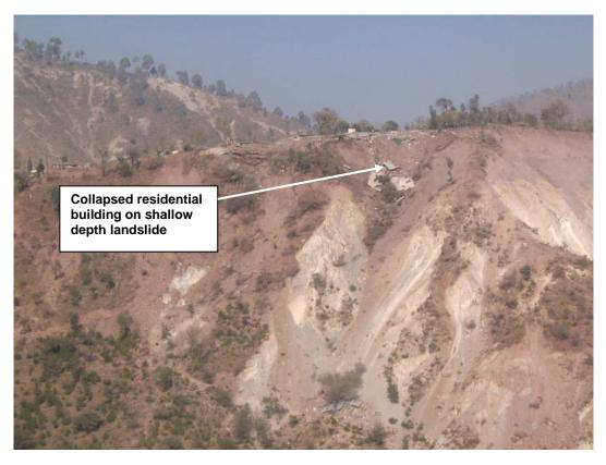
Figure 4.17: Collapsed residential building due to a shallow depth landslide north of Muzaffarabad City
