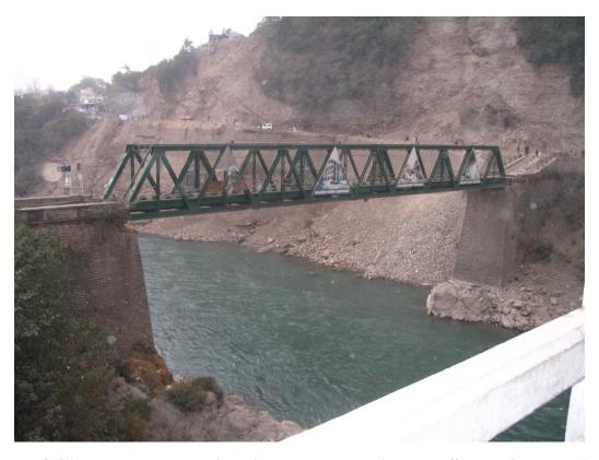
Figure 5.8: Slightly damaged pedestrian bridge across Nelum River, Muzaffarabad. Steel truss single span simply supported on brick masonry abutments
