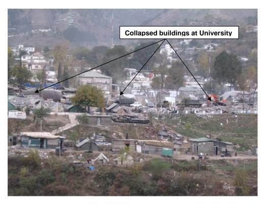
Figure 3.42: Collapsed concrete block URM buildings of the University of AJK, Muzaffarabad
