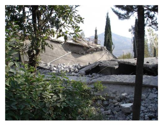
Figure 3.41: Collapsed concrete block URM school building, Muzaffarabad
