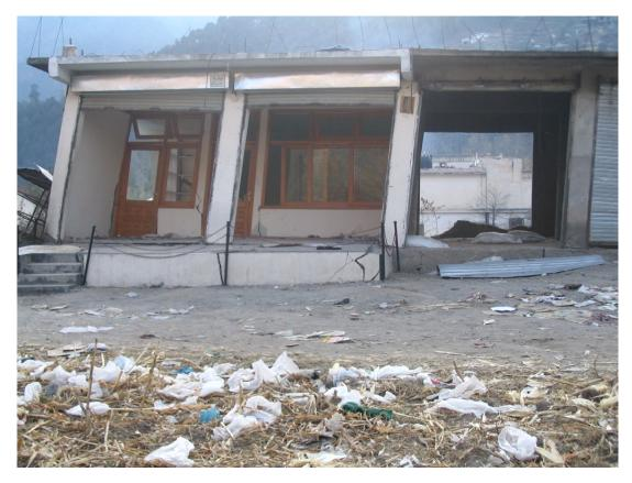
Figure 3.18: Deformed RC frame structure with rotation at the column/slab connection
