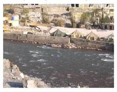
Figure 4.21: Displaced concrete gravity retaining wall by Kunhar River in Balakot
