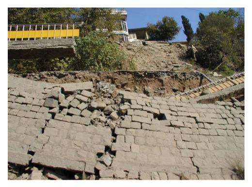
Figure 4.26: Stone block masonry retaining wall in Muzaffarabad, just to the right of Figure 4.25: slippage and collapse of this wall also undermined pavement and road
