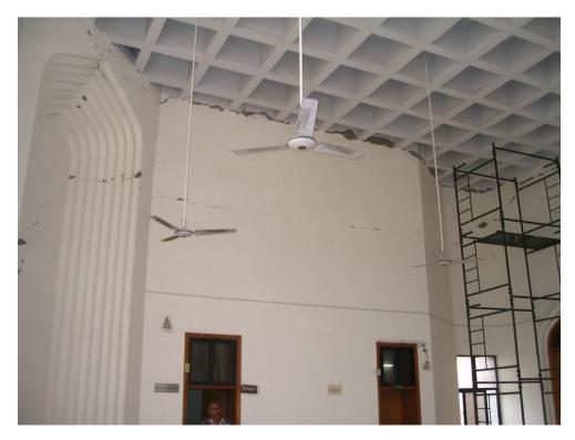
Figure 3.35: Shear cracks through the brick masonry walls of the Muzaffarabad Supreme Court building. Cracking visible at the roof/wall intersection, moderate damage
