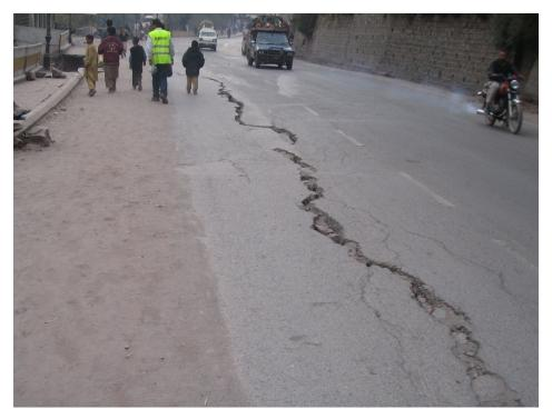
Figure 4.28: Cracks through a major route through Muzaffarabad due to collapsed retaining wall section
