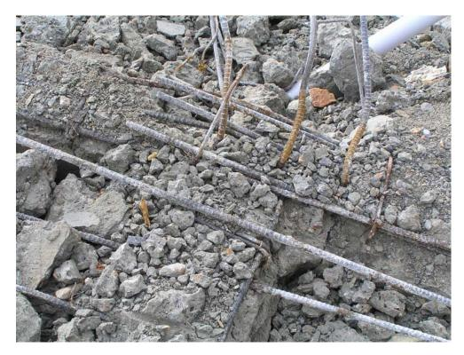
Figure 3.44: Lack of continuity of reinforcement detailing at the beam/column connection
