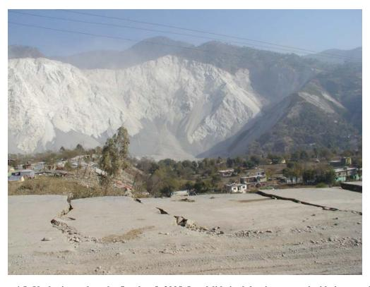
Figure 4.5: Kashmir earthquake October 8, 2005. Landslide in dolomite mountainside just north of Muzafarrabad at Chela Bandi. Also note cracks through road in foreground and damage to buildings in mid-distance
