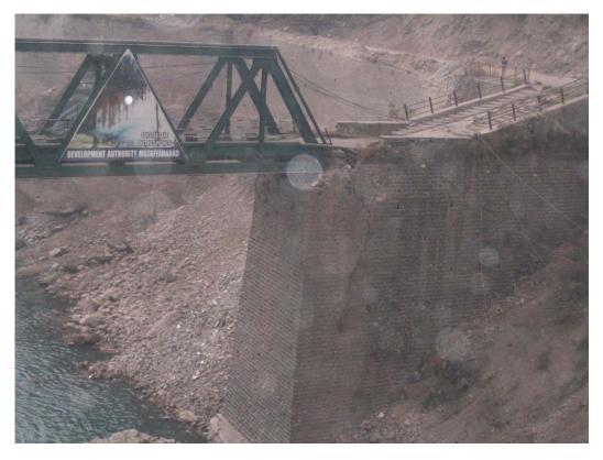
Figure 5.9: Crack at one of the masonry abutments of the pedestrian bridge shown in Figure 5.8
