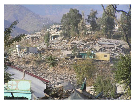
Figure 3.11: Collapsed and extensively damaged concrete block URM residential units on a hill northwest of Balakot city centre (zone 1)
