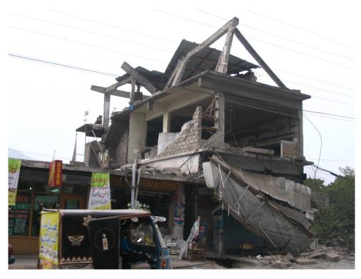
Figure 3.29: Collapsed RC frame of upper floor of 3-storey commercial building with concrete block masonry infill walls. Failure at beam/column connections of upper floor frame, Muzaffarabad
