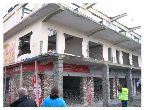
Figure 3.7: Moderately damaged commercial/retail building of RC frame and slab construction with brick masonry infill in Abbotabad
