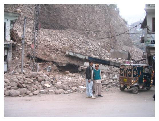
Figure 4.19: Collapsed and buried commercial building from the soil and rock due to the slope failure shown in Figure 4.18, Muzaffarabad
