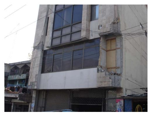
Figure 3.33: Slightly damaged 4-storey RC frame and slab commercial building with concrete block masonry infill, Muzaffarabad
