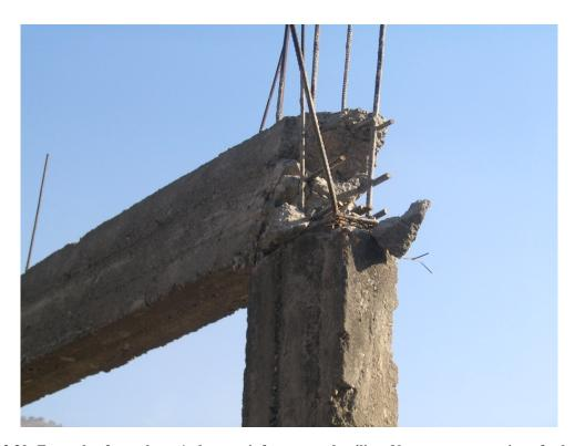
Figure 3.30: Example of poor beam/column reinforcement detailing. No proper connection of column and beam reinforcement for moment resisting action
