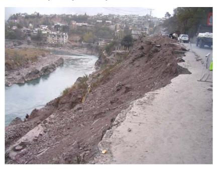
Figure 4.29: Slope failure adjacent to a major route through Muzaffarabad City, danger of further erosion of the road surface
