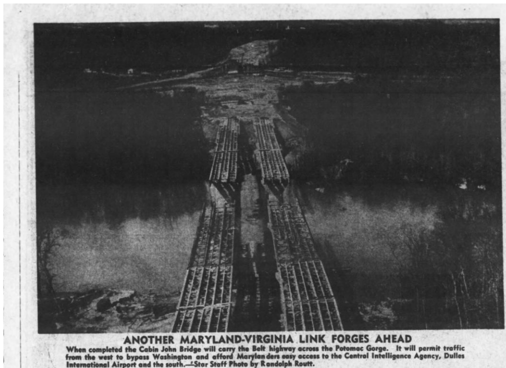
Figure 4.5 Traffic congestion increased due to the Langley project, but it was also a way for the press to measure the movement of CIA staff to and from the site. The ES supported the construction and extension of bridges, such as the Cabin John Bridge because it would alleviate traffic. Source: "Another Maryland-Virginia Link Forges Ahead," ES , May 4, 1962, p. 75.
