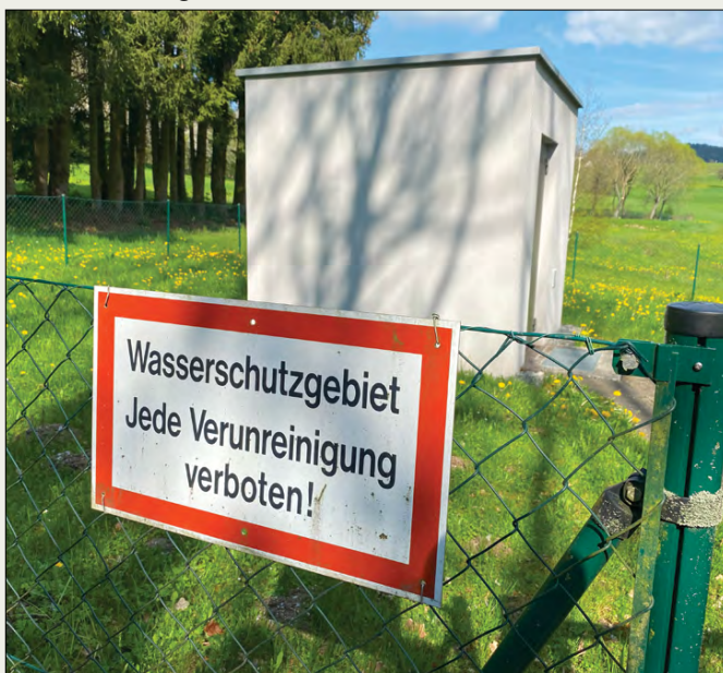
'Water conservation area - any pollution prohibited!' Source protection measures around a borewell source for the WWG St Oswald co-operative. Drinking water sources have ascending zones of protection in Austria.
