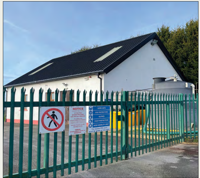
The Killanny & Reaghstown GWS water treatment plant. The GWS is one of nine GWSs in the Monaghan DBO bundle.
