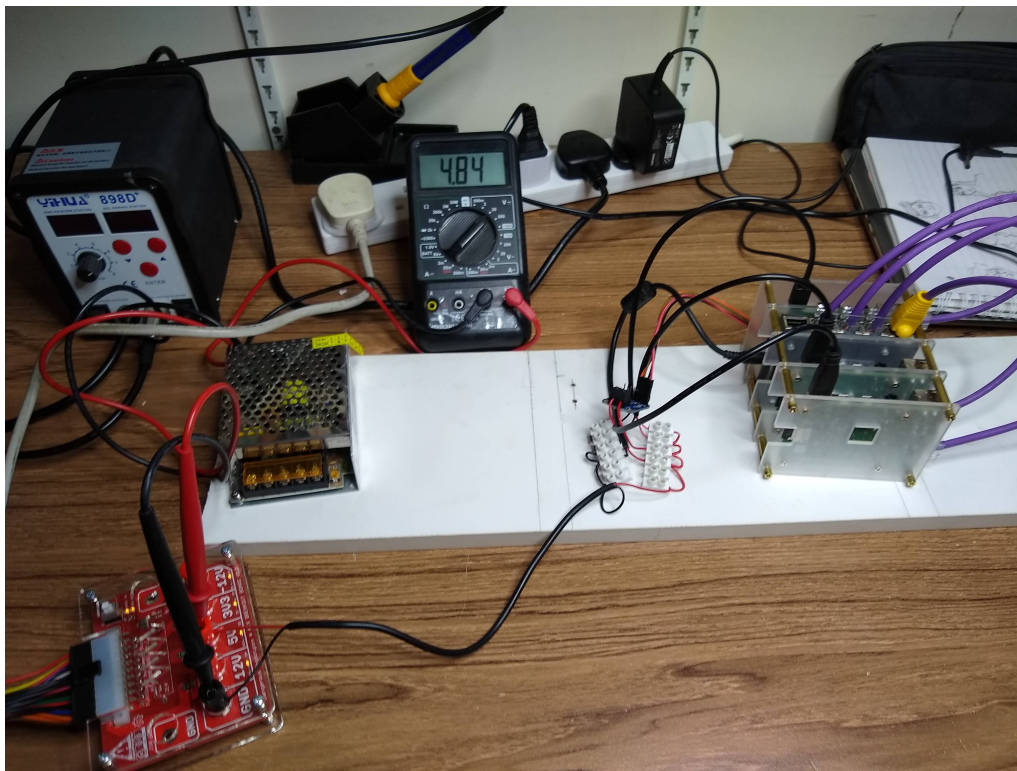
Figure 5.4.1: Voltage verification using a multimeter
